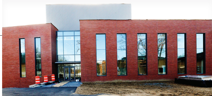
Skidmore is nearing completion of the first phase of the Center for Integrated Sciences.
